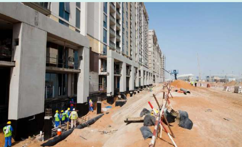
Pipe installation in 2010
