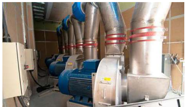
Centrifugal fan – Create high volume of airflow up to 25 m/s.
