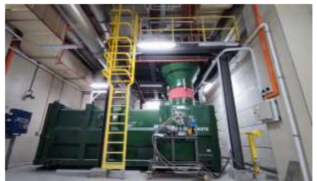
Compactor container – Larger load of general & recyclable waste collected into air-tight sealed container.
