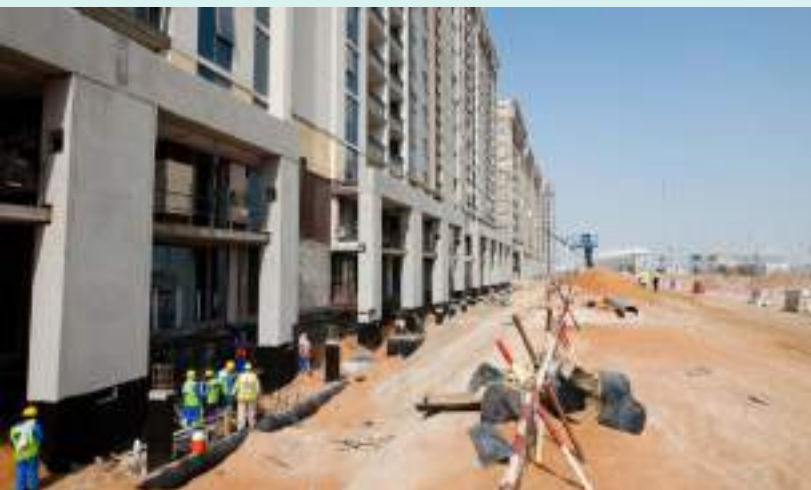
Pipe installation in 2010
